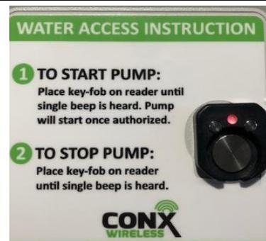
**Step 3 – Turn Pump Off, Check Email for Receipt:** To stop pump, place key-fob on reader until single beep is heard and the red light on the reader is no longer visible. Your transaction has been completed. Please check your email for transaction receipt.
